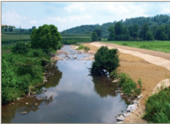
Figure 9.1a Restoration site immediately after construction.
