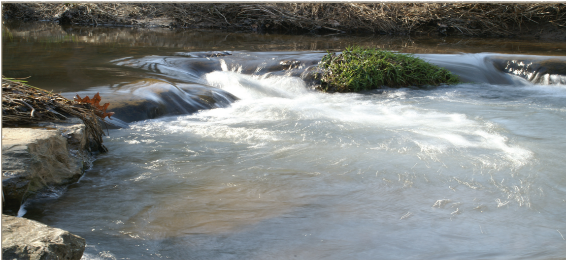
FIGURE 9.2 FLOW TURBULENCE CREATED FROM ROCK CROSS VANE STRUCTURE
